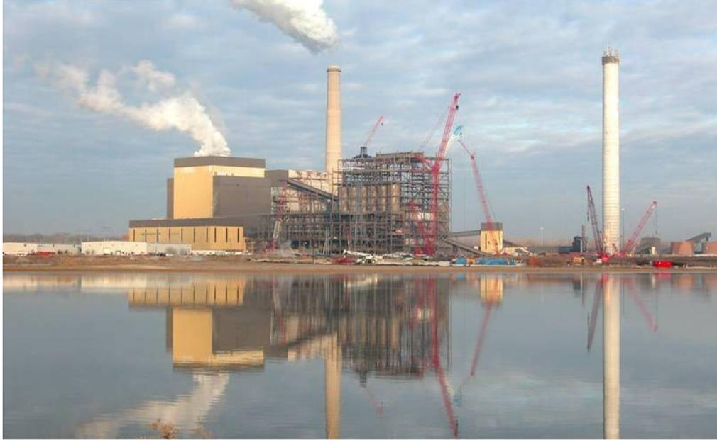
The boiler top girders, a major milestone for a sliding pressure Benson type boiler, were set in February 2005. With these in place, the boiler proper erection work began. At the same time, other mechanical equipment (Condensers, Coal Mills and etc.) was installed. The crossover coal conveyor between Units 3 and 4 was ground assembled and lifted into place in May 2005.
