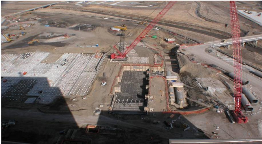
Structural steel and ductwork delivery began in May 2004. One of the integral aspects of the delivery plan was the use of the Missouri River and, as such, a temporary barge unloading facility was constructed by the summer of 2004. This allowed for module shipments including box sections of boiler ductwork.
