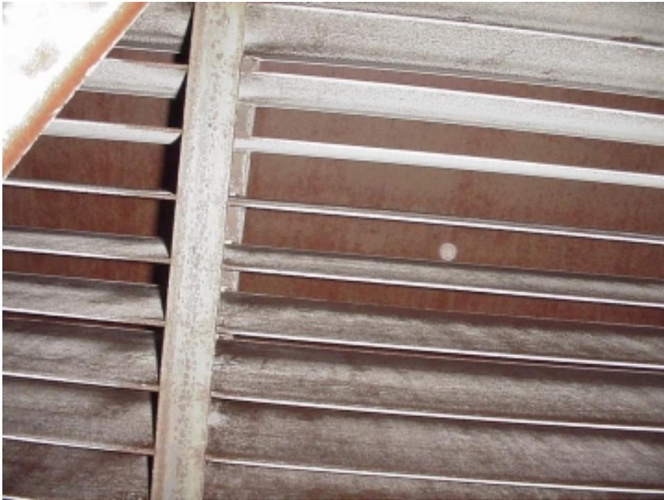
Plate 2: SCR Inlet Turning Vanes
