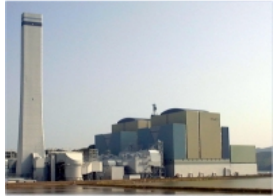
Fig.3 Tachibanawan Thermal Power Station
