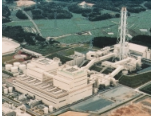
Fig.1 Haramachi Thermal Power Station, Unit No.2
