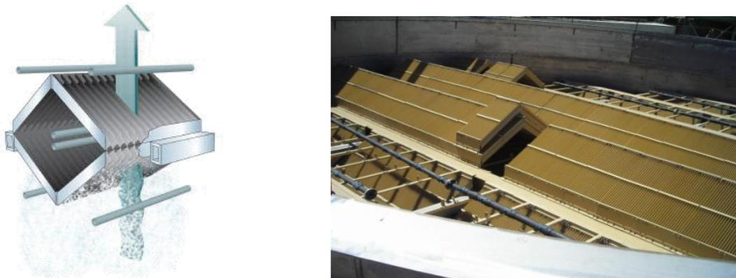
Fig. 11 Mist Eliminator Arrangement
